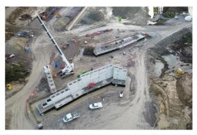
Precast concrete bridge abutments are installed at Station Road
